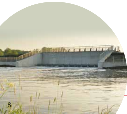
The innovative combination sluice of Bergenmeersen
