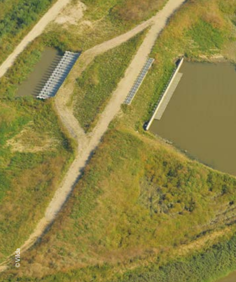
outlet construction at the overflow dike
