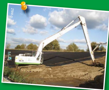
overflow dike under construction
